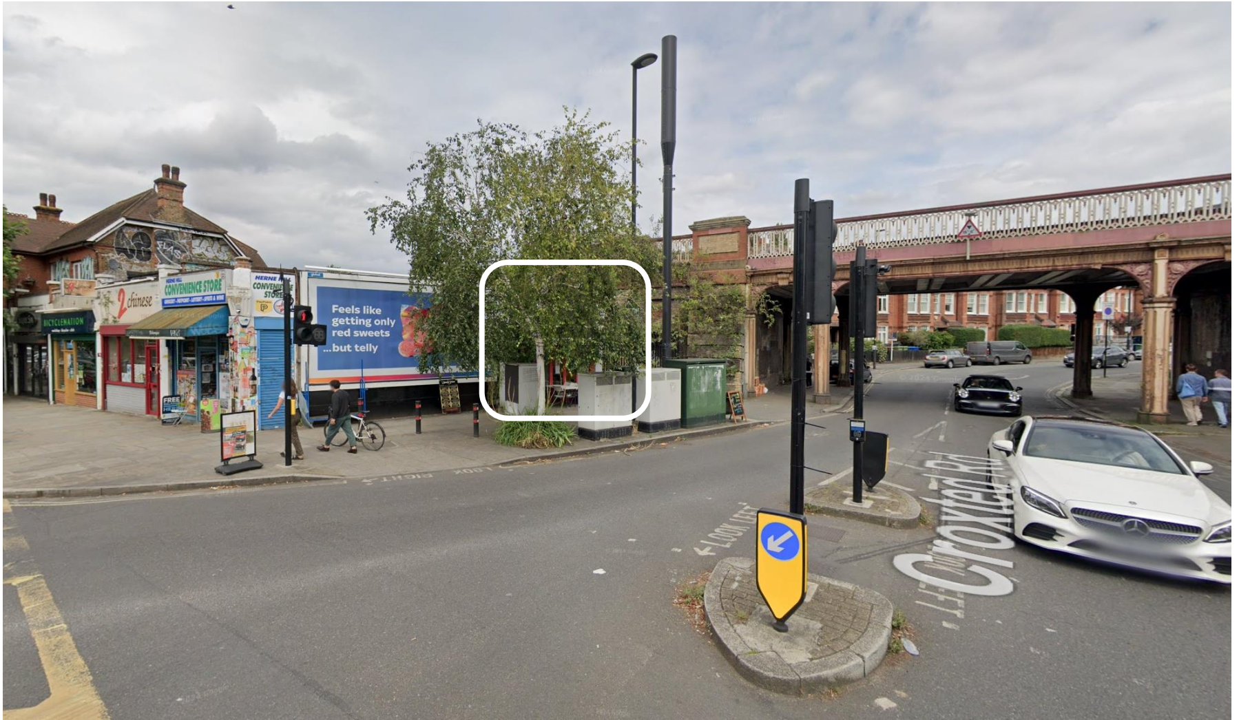
Location of telecoms equipment outside 294 Croxted Road, SE24 9DA
